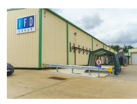
The 150m2 area was excavated by our team on site, who then installed and compacted a crushed concrete sub base, which was subsequently covered with the poured concrete you can see at finish level.
