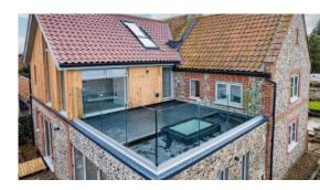
The biggest challenge with the superstructure was the detail where the flint external skin wrapped around the back right corner. To do this we had to use stainless steel trims to form an end point to both the side and rear wall that we could run the flint work up to and this process was repeated around window and door openings also.
